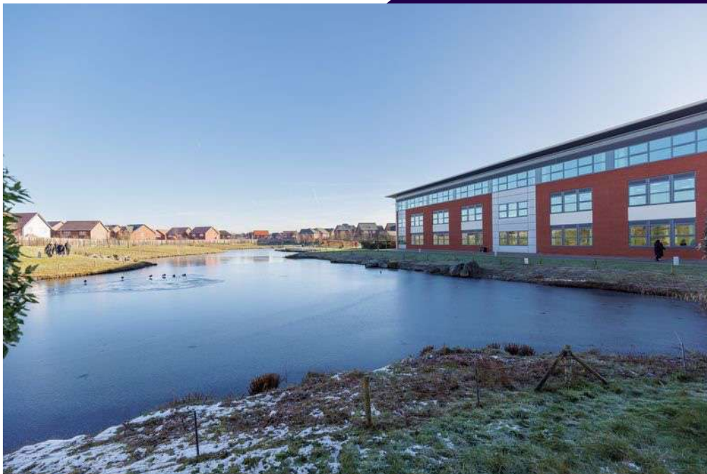
CLEARWATER 4, LINGLEY MERE BUSINESS PARK
